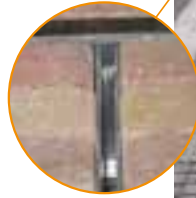
Integral lifting key
